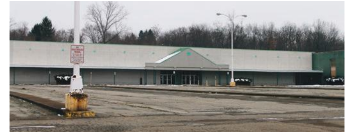
Figure 6.21 - The former McGuffey Plaza in 2013.
