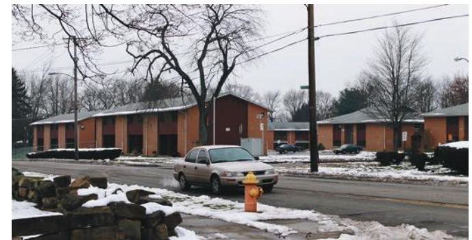
Figure 6.26 - Plaza View Apartments, near McGuffey Road.
