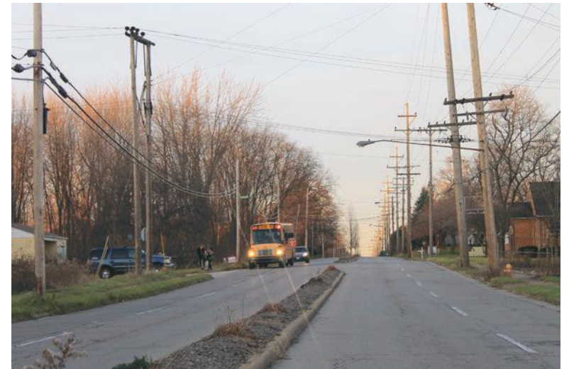
Figure 6.58 - A small median divides lanes of traffic on Jacobs Road.
