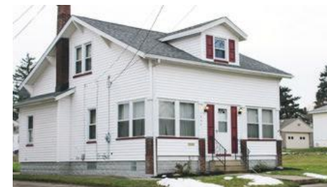
Figure 8.40 - Nearly all houses were built before 1979.
