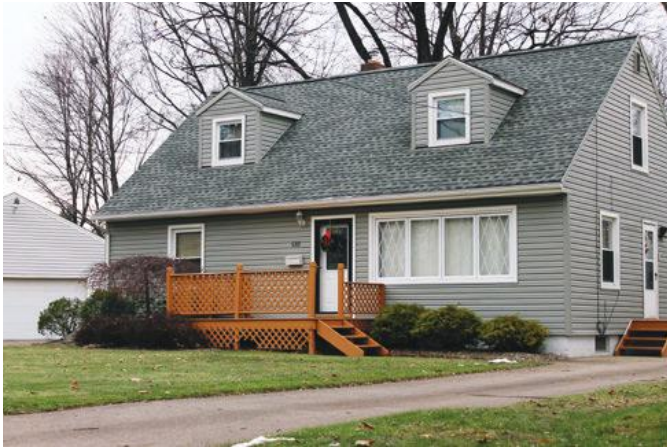
Figure 8.14 - Nearly 75% of homes were built in the 1950s and 1960s.
