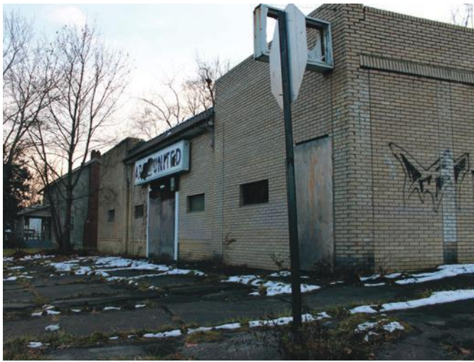
Figure 9.39 - Vacant structures line Logan Avenue.
