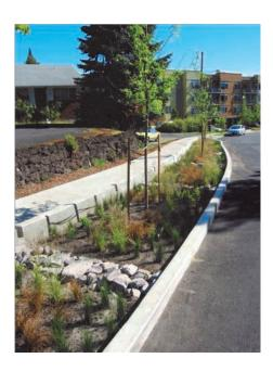
Green infrastructure treatments in Portland, Oregon, clean and manage stormwater on site using native plants and appropriate slope design.
